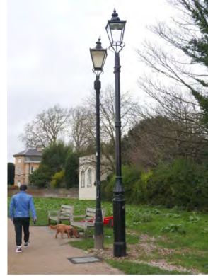
LH An original cast-iron 'Revo' column (fitted with a modern repro-Victorian lantern and box) on the LH side with a newly installed, mild-steel, repro-Victorian column and lantern alongside of significantly increased height and girth - also showing the backfilled trench for the new, below-ground electricity supply.
