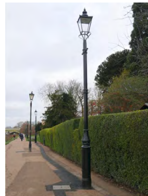
Views along Cholmondeley Walk downstream and upstream showing the failure to reinstate the attractive, bonded-gravel surfacing after the excavation and back-filling of a trench for the new electrical supply.
