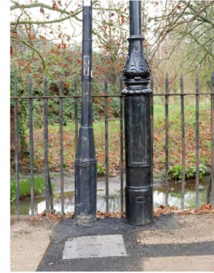
LH An original cast-iron 'Revo' column (fitted with a modern repro-Victorian lantern and box) on the LH side with a newly installed, mild-steel, repro-Victorian column and lantern alongside of significantly increased height and girth - also showing the backfilled trench for the new, below-ground electricity supply.
