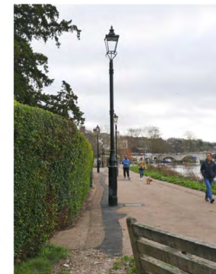
Views along Cholmondeley Walk downstream and upstream showing the failure to reinstate the attractive, bonded-gravel surfacing after the excavation and back-filling of a trench for the new electrical supply.
