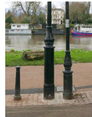
LH One of the newly installed repro-Victorian columns of increased height and girth on the LH side with one of the relatively recently installed repro-Victorian, standard 'Oxford' columns (as recommended in the Council's own published guidance for use along the riverside) alongside, at the river end of Old Palace Lane by the grade I listed Asgill House,
